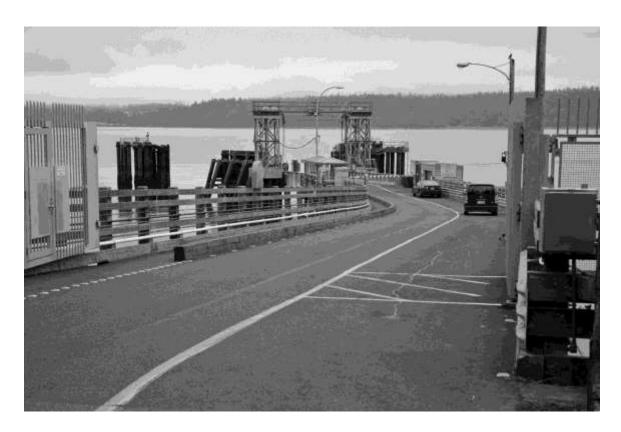
The current photograph shows the dock in 2009 with the security gate installed after 9/11, a significantly expanded passenger shelter moved to the left side, and expanded storage for ferry equipment on the right. The dock is significantly wider and a walk-on passenger walkway was added on the left side of the dock.
