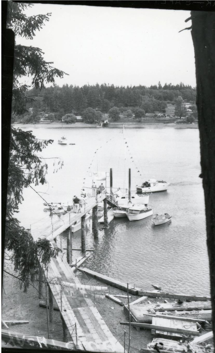
The original photograph taken in the early 1950s shows the dock with the dogleg to the right and the ramp down to a float. These features are still basically the same. The bulkhead is also still basically the same except that now it is hidden under the deck that is cantilevered out over it. The original photograph shows one sailboat, all the other boats are powerboats from about 15 to 30 feet in length. Today the club is 35% powerboats and 65% sailboats ranging from 22 to 65 feet in length.
