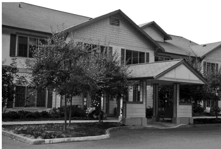
Vashon Community Care Center 2009
