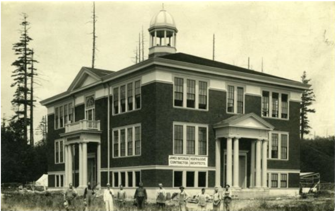
Vashon High School under construction: courtesy Vashon-Maury Island Heritage Museum
